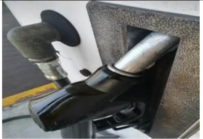
Nozzle leaking needs repairs
