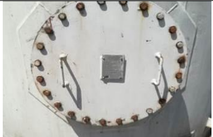
Rusted manhole bolts
