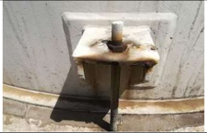
Rusted tank anchor
