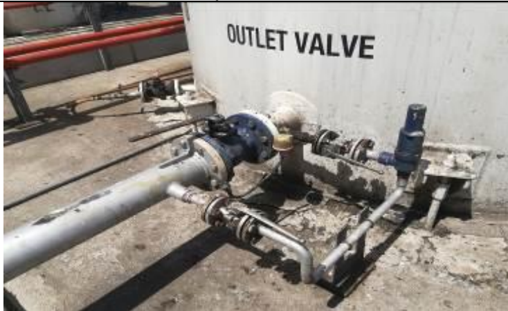
Tank thermal relief
