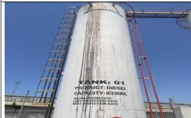
Tank 1 visible spillage
